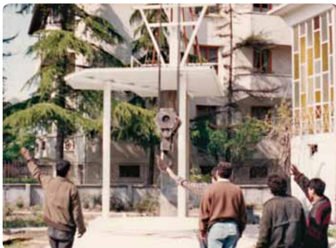
■ The crane lifts the dish in place
