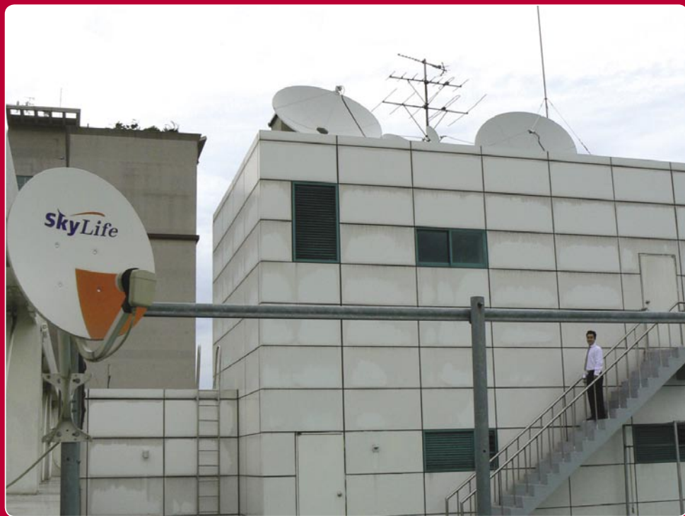
David Choi on the roof of the Topfield building. A small antenna can be seen to the left for the reception of SkyLife on KOREASAT along with other antennas
